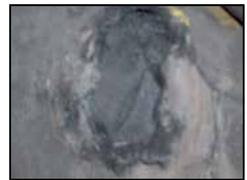
Melted or Charred areas
